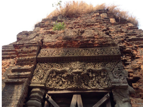
Figure 5 Finely carved pediment on remaining tower.
