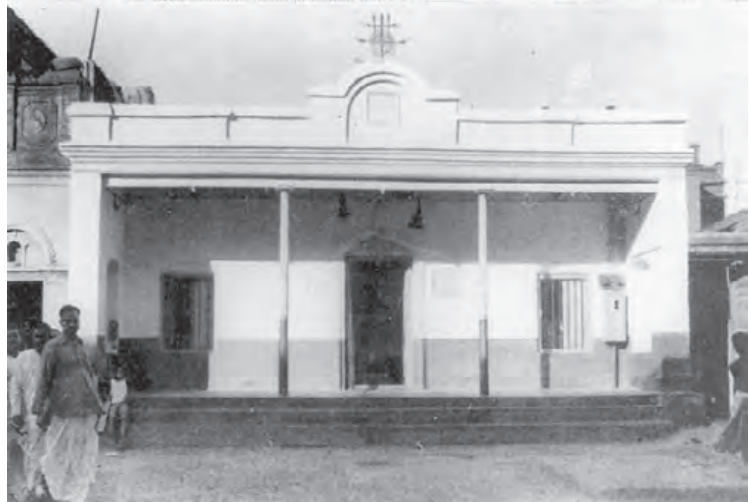
Ramkumar's Sanskrit School at Jhamapukur
